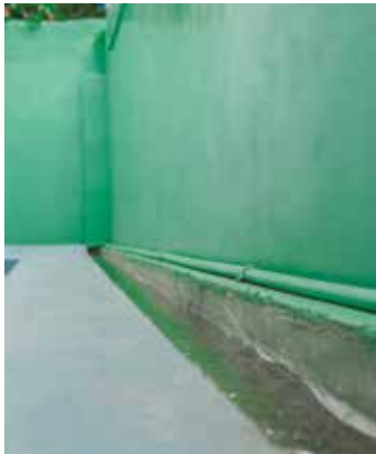
Photo 8: Drainage with slope
