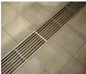
Photo 9: Drainage with rat-proof entry
