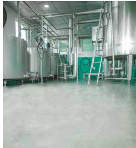
Photo 1: Example of a non-absorbent factory floor
