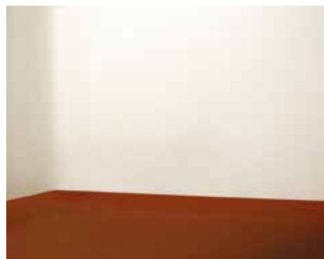
Photo 2: Light-coloured wall, washable, non-absorbent, easy to clean and disinfect
