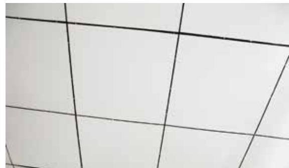
Photo 6: Solid, light-coloured and easy-to-clean ceiling
