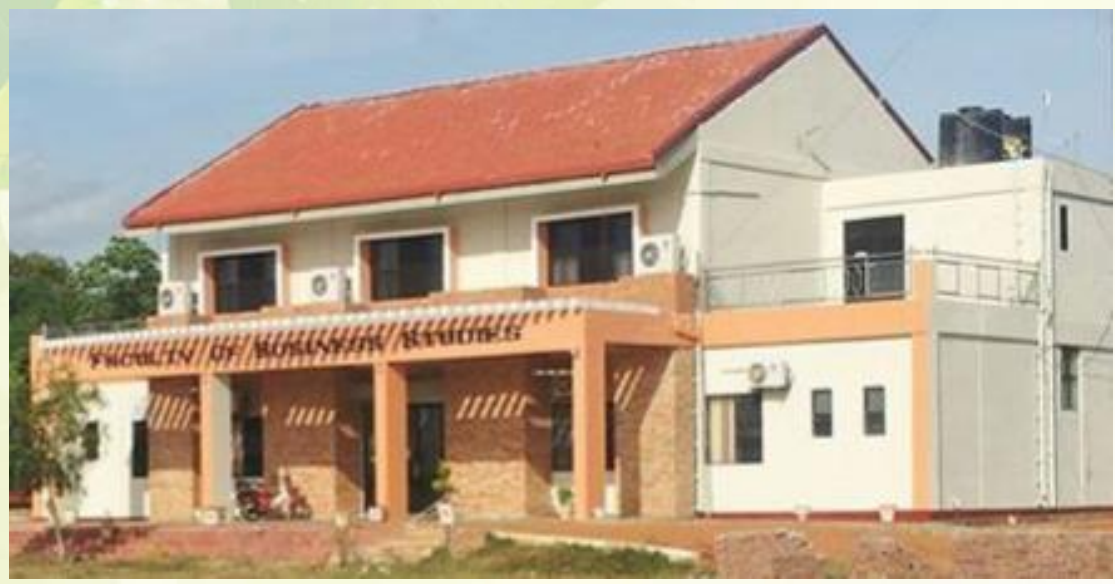
EXISTING FACULTY OF BUSINESS STUDIES BUILDING
